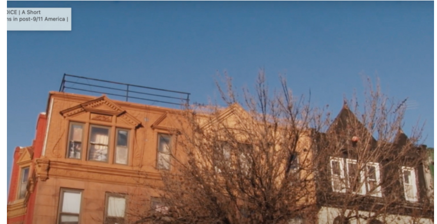
Outside my house on S 8th Street - my living room is under that arch.
